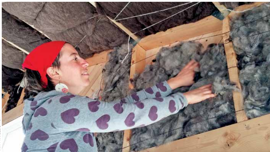
■ Jessie Litven is building her tiny house in Halifax's north end. Among her resourceful innovations is the use of PEI-milled sheep's wool for insulation.
